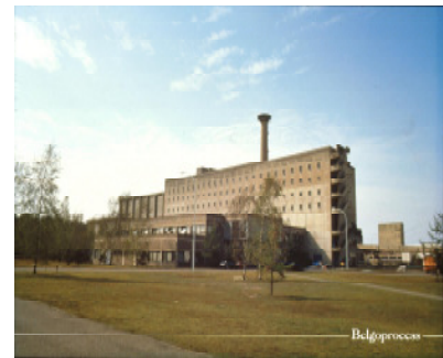
Figure 3. Main process building of the former Eurochem reprocessing plant
