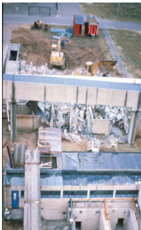
Figure 1. Demolition of buildings 6A/6B
