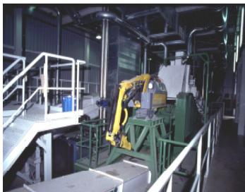
Figure 4. General view of the concrete crushing and sampling facility
