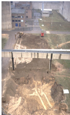
Figure 2. Green field conditions after demolition of buildings 6A/6B
